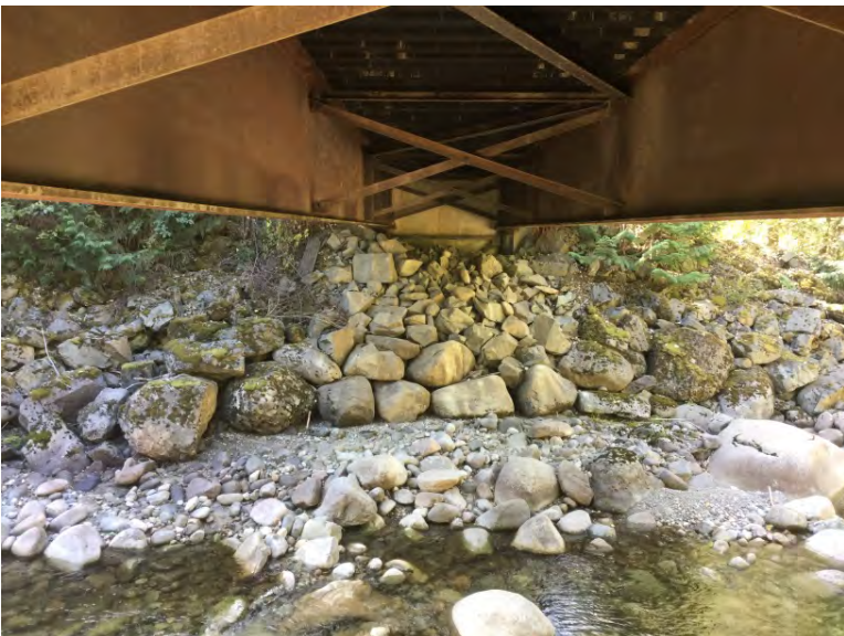
Left Bank Abutment when facing downstream
