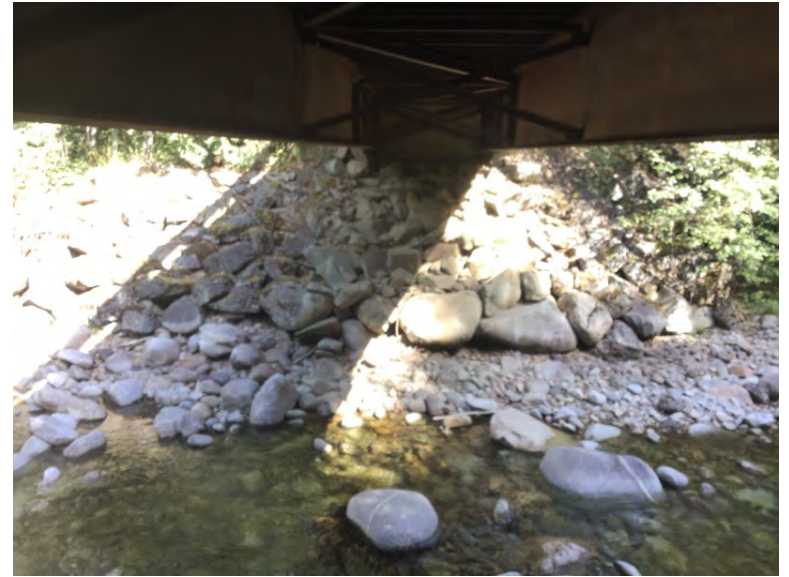
Right Bank Abutment when facing downstream
